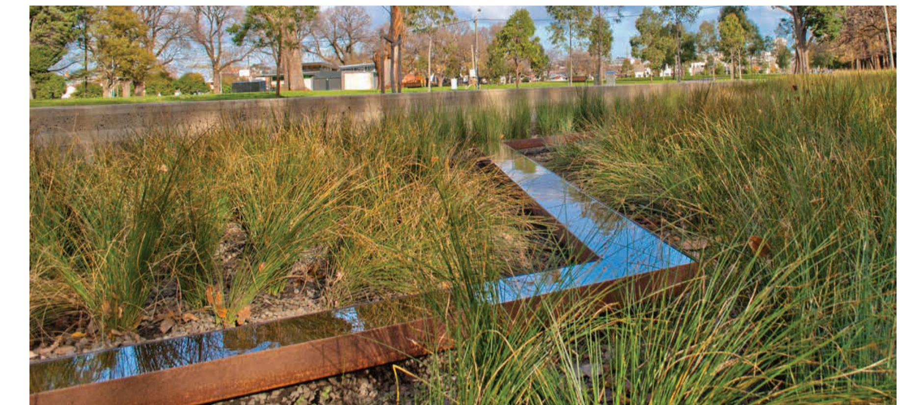
Narrower channel sections will create faster flowing, noisier water.
