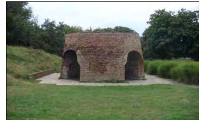
THE LISTED LIME KILN
